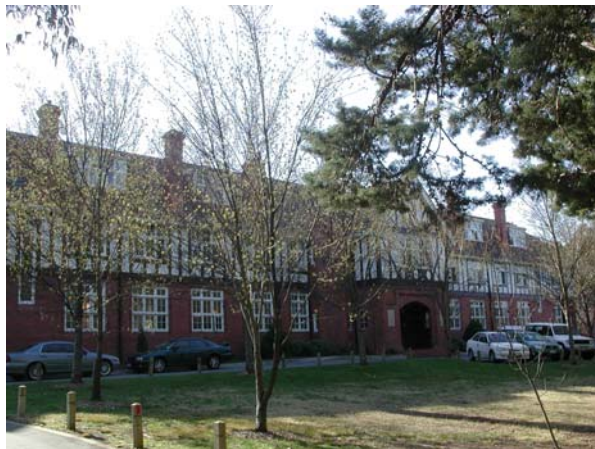
Figure 7. CEGGS Boarding House from north east (EMA 2004)
