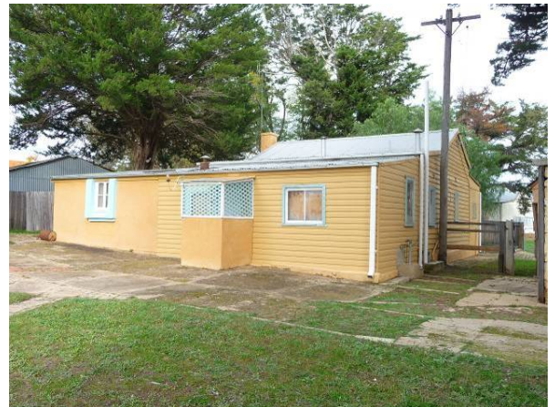
Figure 5 North and west facades (ACT Heritage, 2014)
