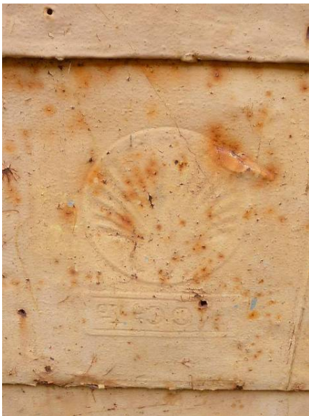
Figure 12 B.I.O. Shell kerosene tin cladding on western shed (ACT Heritage, 2014)
