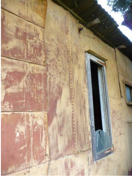
Figure 11 Tin cladding on east laundry facade (ACT Heritage, 2014)
