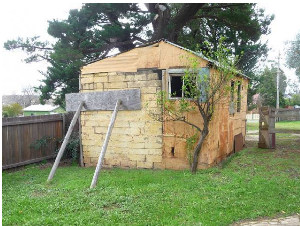
Figure 8 Southern end of western shed and laundry (ACT Heritage, 2014)
