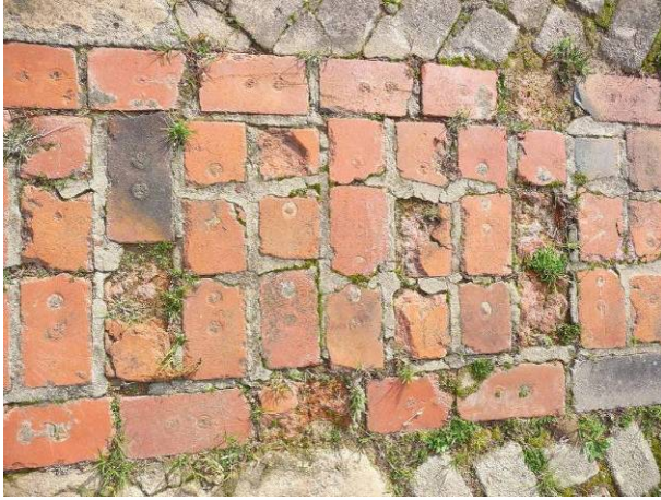
Figure 15 Brick paving (ACT Heritage, 2014)
