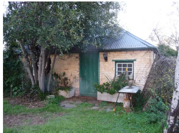
Figure 8 The Oaks external kitchen east facade
