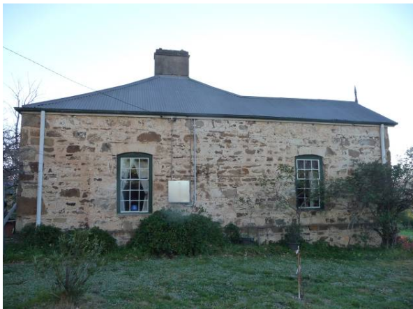
Figure 6 The Oaks east facade (ACT Heritage, 2014)
