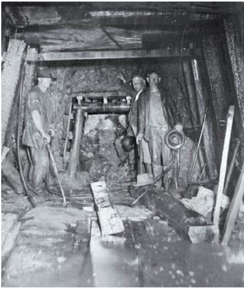
1927 – Construction of the main outfall sewerage tunnel. Photo shows the joining up of two tunnels, possibly under old Westlake. Many of the tunnel workers came from mining towns such as Captain's Flat, Araluen and Major's Creek. Photo by permission of the National Library of Australia.
