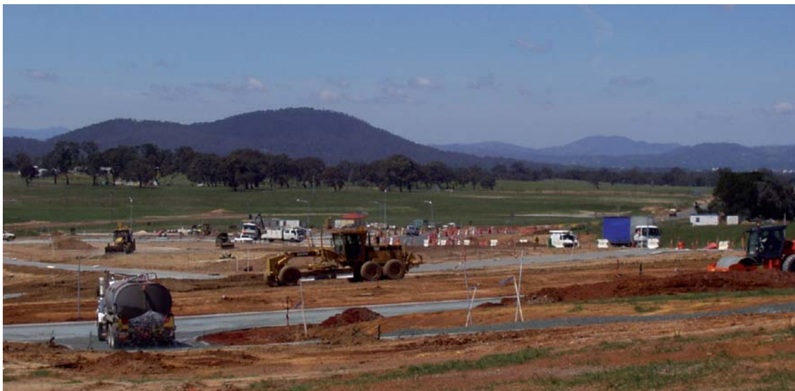
Above: Civil works at Horse Park 2 Housing Estate
