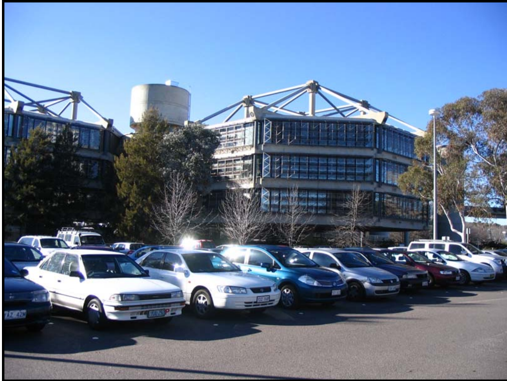
Callam Street entrance view of the Callam Offices:
