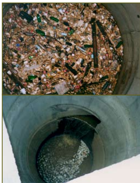
A proprietary GPT unit: (i) full of urban litter, and (ii) after cleaning
