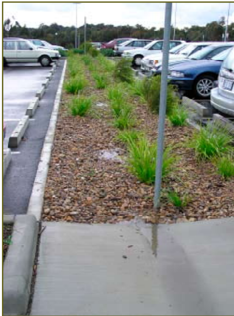
A car park bio-swale
