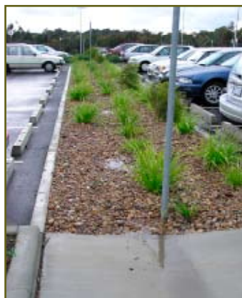
Bio-swale drainage system
