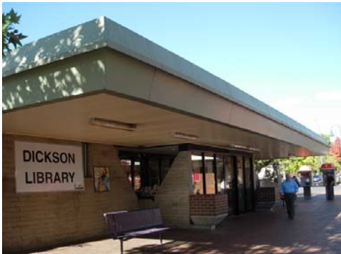
Figure 9. Dickson Library, S side - entrance (Truscott 10/4/08)
