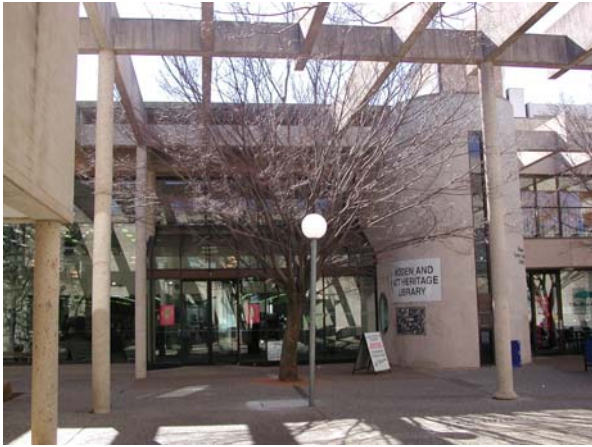
Figure 4. View toward Entry (EMA 2004)
