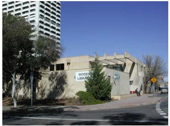
Figure 7. View from NW (EMA 2004)
