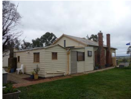
Callum Brae Homestead The original two-roomed building is at the rear.
