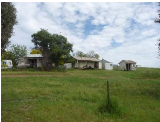
1920s/1930s shearer's quarters including sleeping quarters, kitchen, and shower room.
