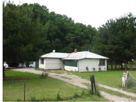
1950s station-hand's cottage
