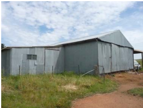
1970s machinery shed
