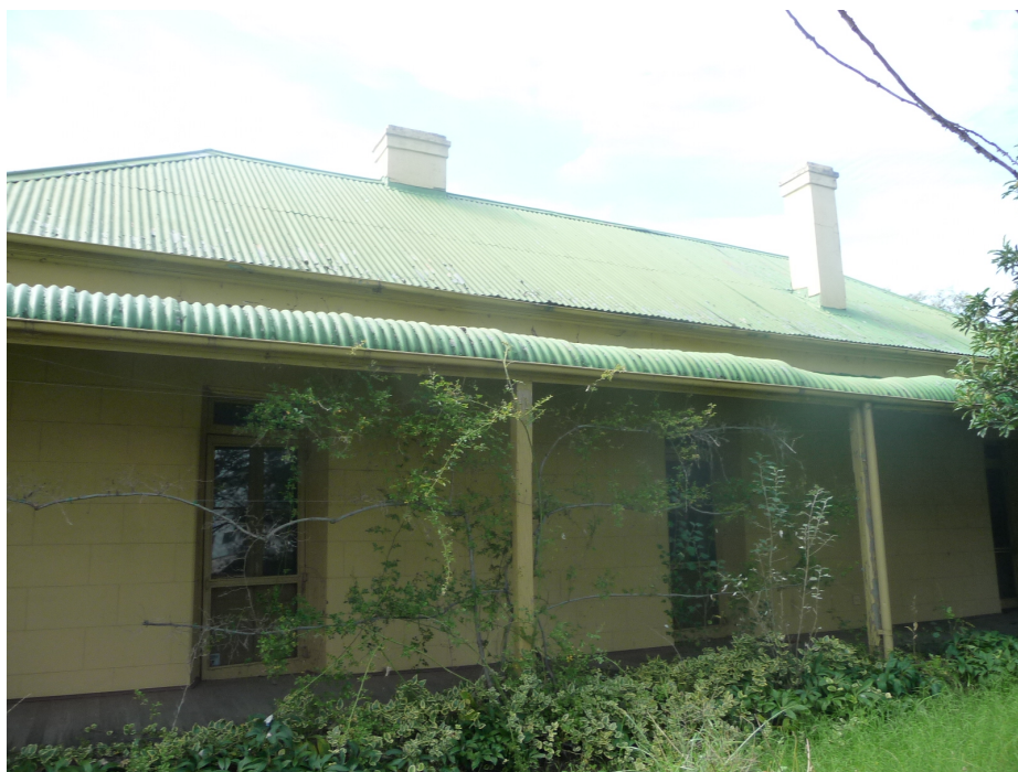
Fig 3: Pisé homestead with bull-nosed verandah, c 1909
