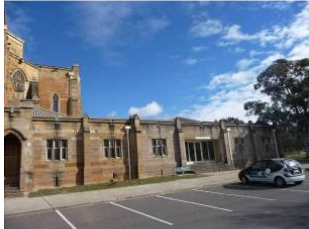
Image 3. Hall northeast facade. (ACT Heritage Unit, 2013)
