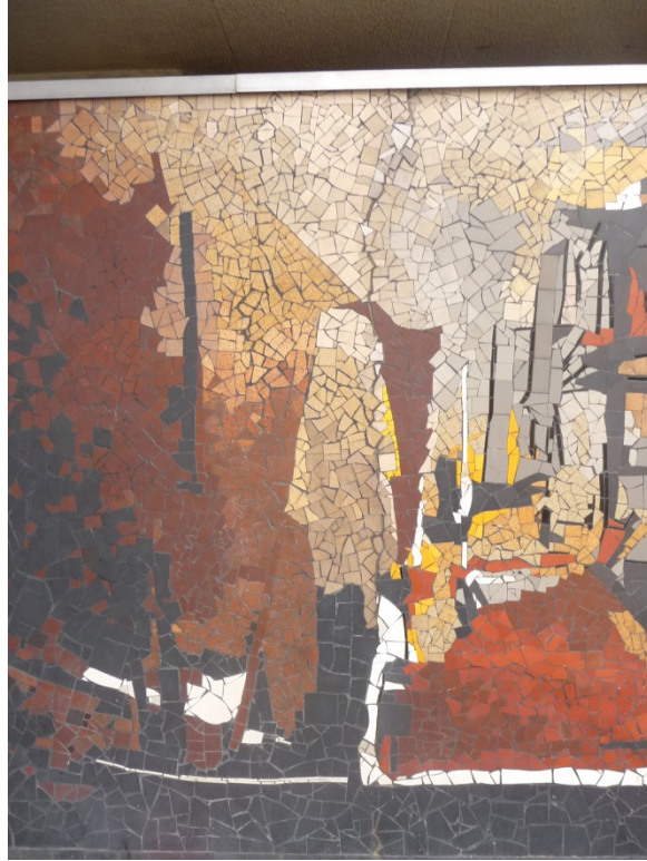
Figure 4. Repaired Structural Crack 1, situated in sections 5 and 6 (ACT Heritage Unit, Sep 2012).
