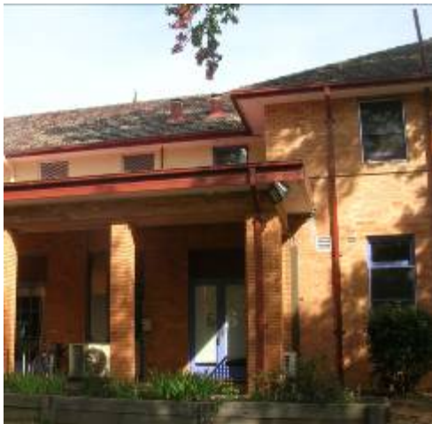
Image 10 Detail of brickwork to north verandah 22 April 2014 (Source: ACT Heritage Unit)
