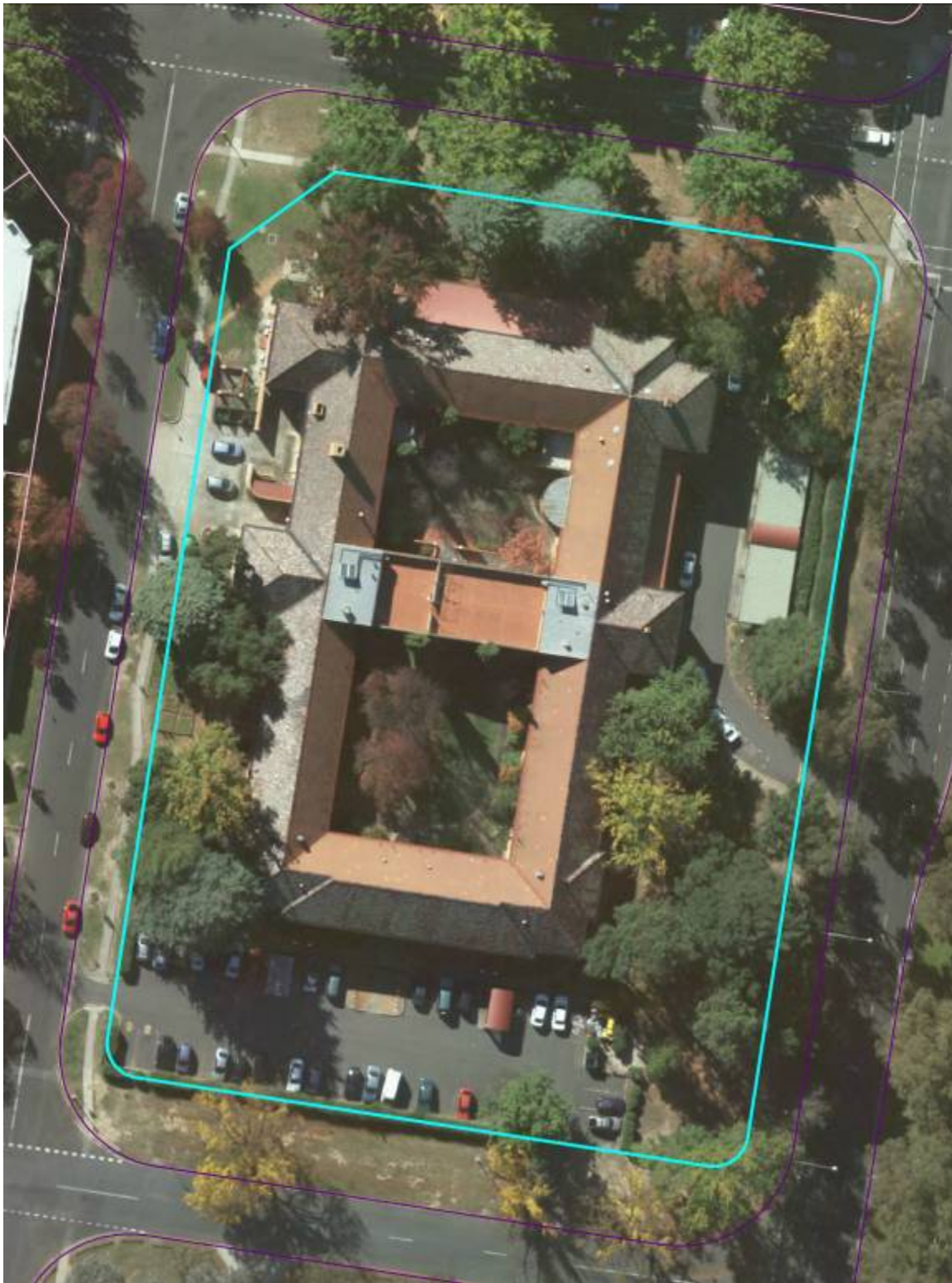
Image 1 Provisional Registration Boundary, Havelock House (Aerial imagery accessed May 2014).
