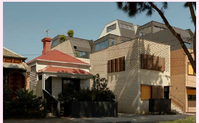
Photo 13: 6 2 Barry St, Brunswick VIC, Fieldwork. Photo: Tom Ross
